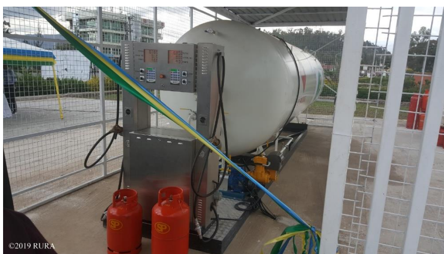
Figure 26:SP LPG Skid in Musanze District(storage and filling unit)
