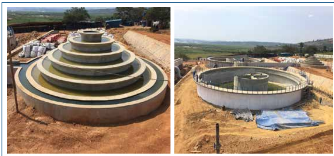
Figure 48: The progress of construction works: Cascade Aeration and Clariflocculators
